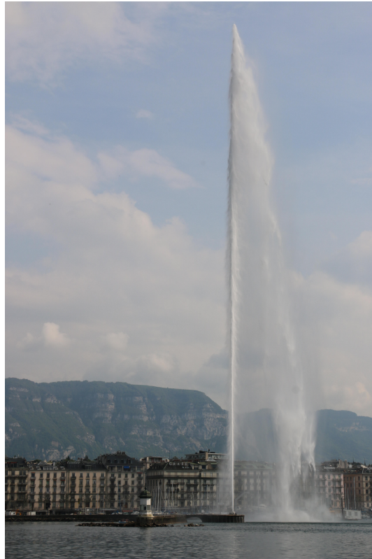
Fig. 2.18 The Jet d’Eau, the famous symbol of Geneva, Switzerland, the hosting city of the CERN laboratory. The water fountain has its origin in a safety valve for a hydraulic power network from 1886. In its nowadays form as a landmark and tourist attraction it reaches a height of 140m, for which 500 litres of water per second are ejected at a speed of 200km/h.
